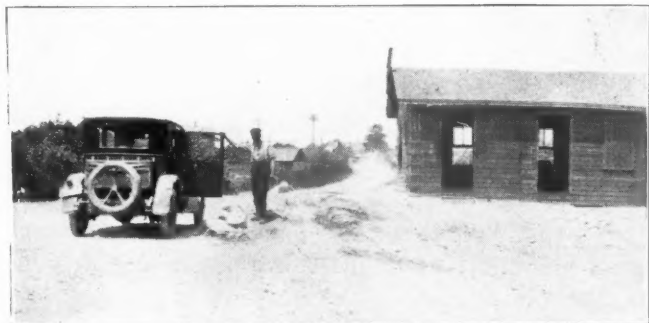
Office and Weighing Platform
